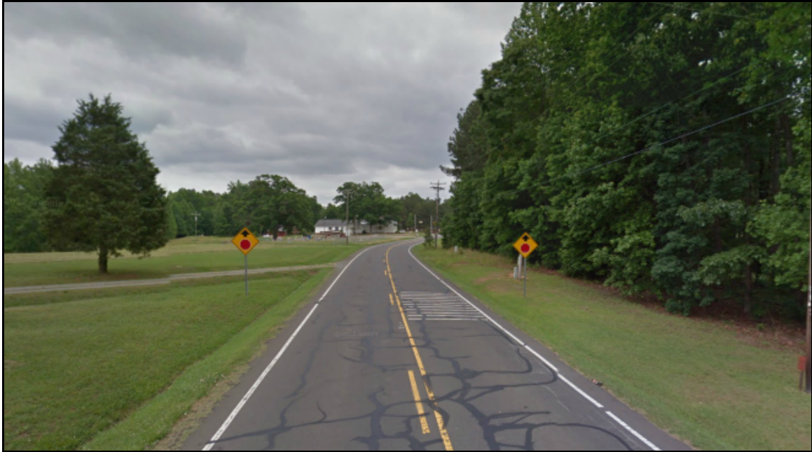
Google Maps (May 2012) – Stop Ahead Warning Signs and Rumble Strips on Southbound NC 96 Approach
